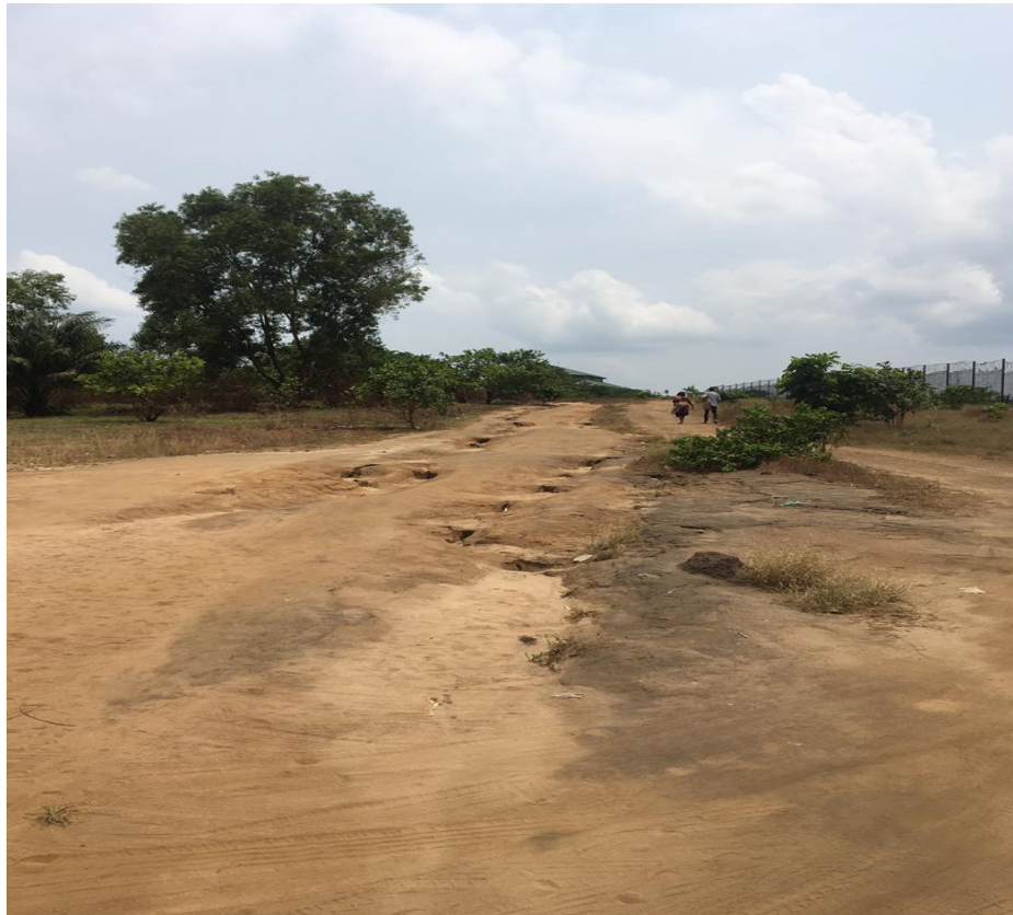
Figure 5: Rill Erosion by UNIUYO Post Graduate School
